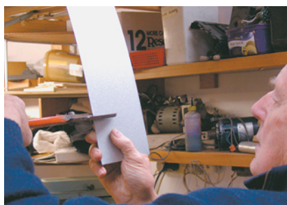
Cut the flashing.
